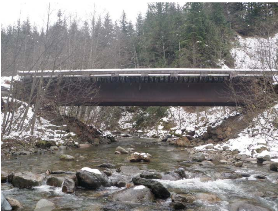
View from downstream.
