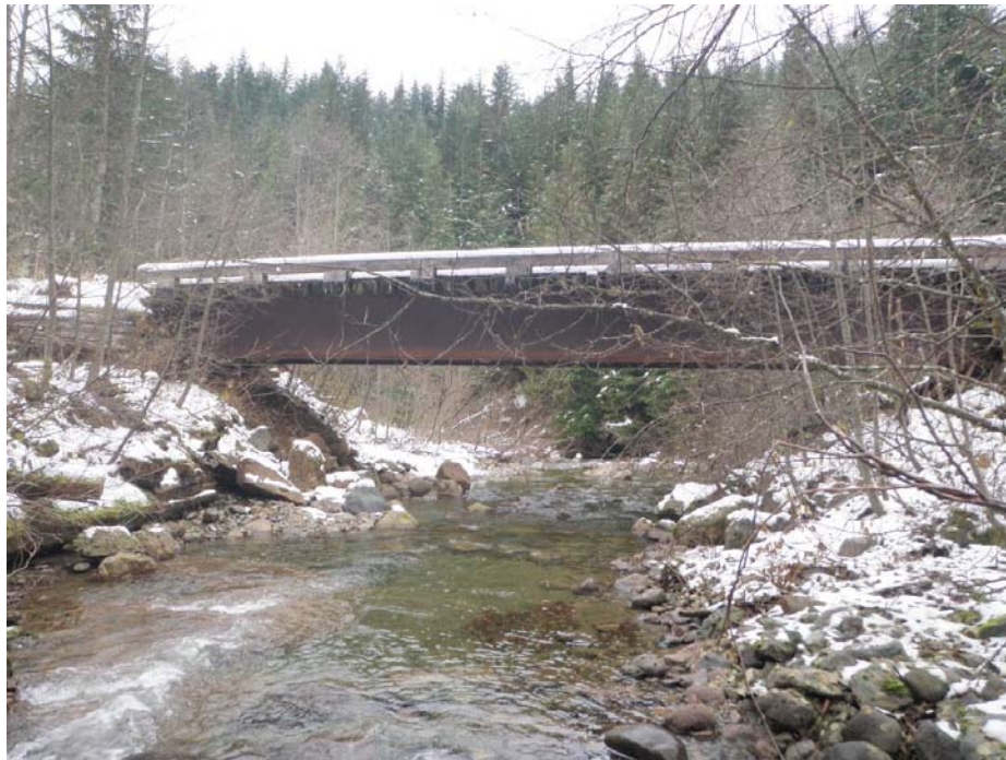
View from upstream.
